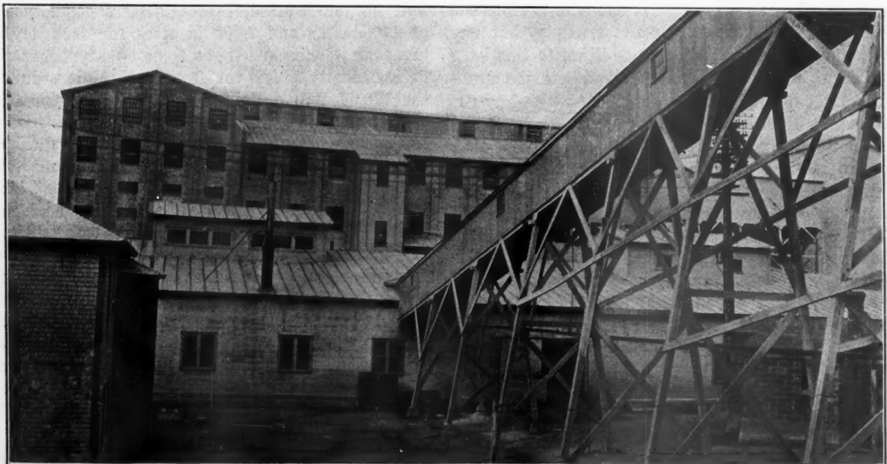
View of Mill with Conveyor in Foreground Which Runs to Bins from Which Waste is Loaded into Cars for Waste Dump
